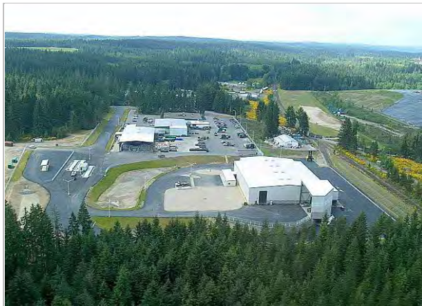
Olympic View Transfer Station
