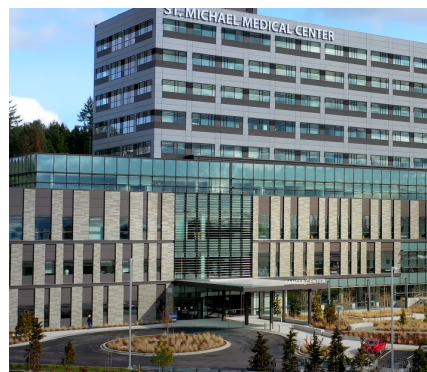
Figure 3.23 St. Michael's supports Silverdale's position as a growing regional medical hub
