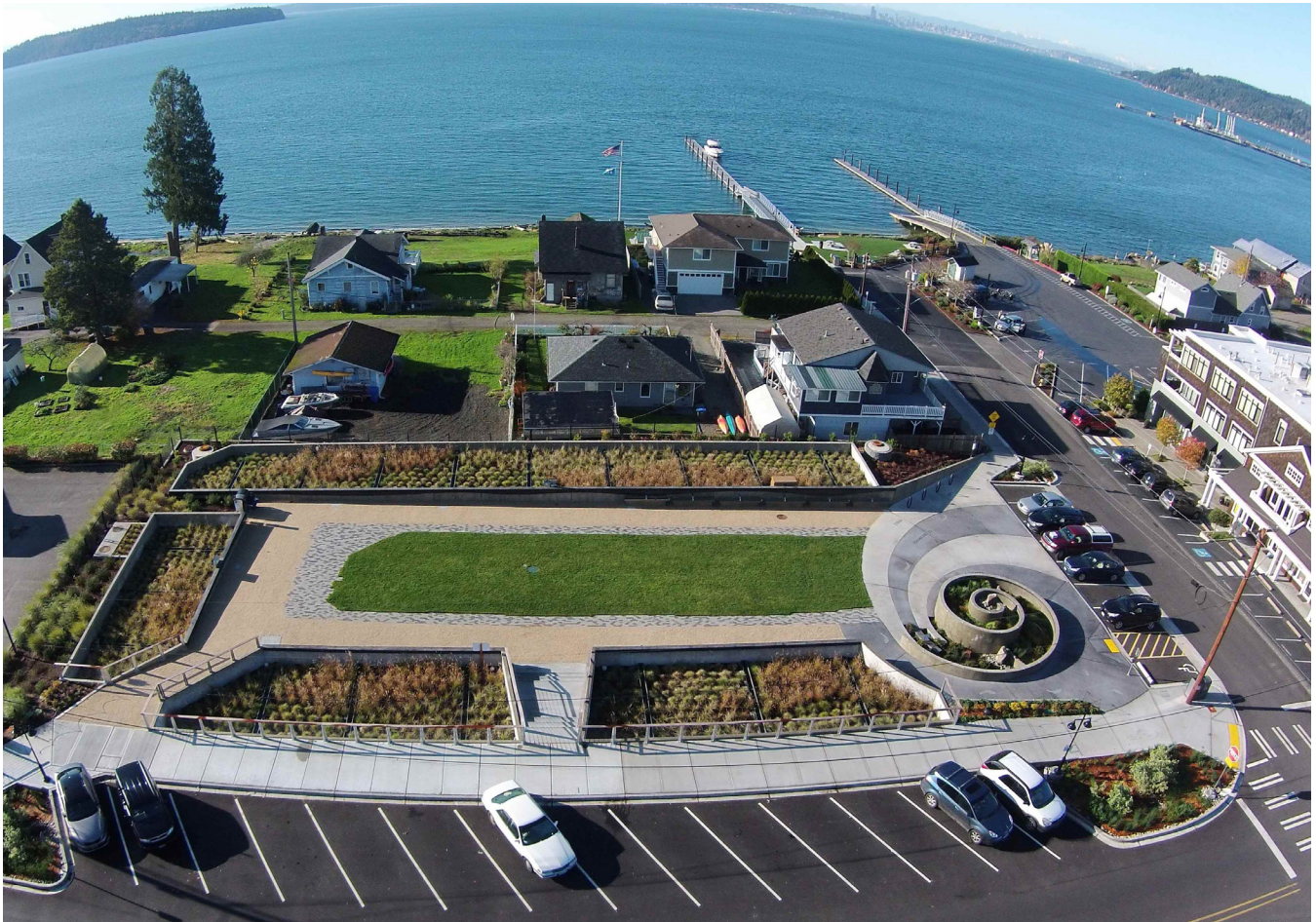
Figure 6.39 Manchester Stormwater Park treats stormwater from roads, parking lots, and residential and commercial properties in the small Kitsap County community of Manchester
