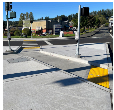
Figure 6.27 Improvements to pedestrian infrastructure on Silverdale Way
