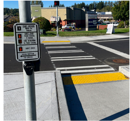
Figure 6.33 Pedestrian safety infrastructure on Silverdale Way
