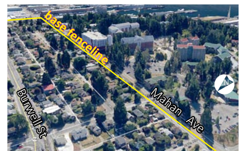
Figure 4.2.4. NBK-Bremerton perimeter context near the Naval Gate (looking southeast) (image credit: Google Earth)
