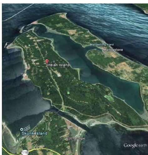
Figure 4.2.18. NAVMAGII's island setting necessitate good coordination with surrounding communities on infrastructure and utilities.
