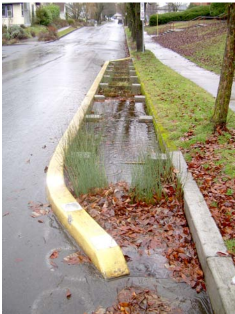
Figure 4.5.5. Example of green stormwater infrastructure emulating natural drainage, where carefully chosen plants and soils treat stormwater runoff and allow infiltration to reduce water pollution.
