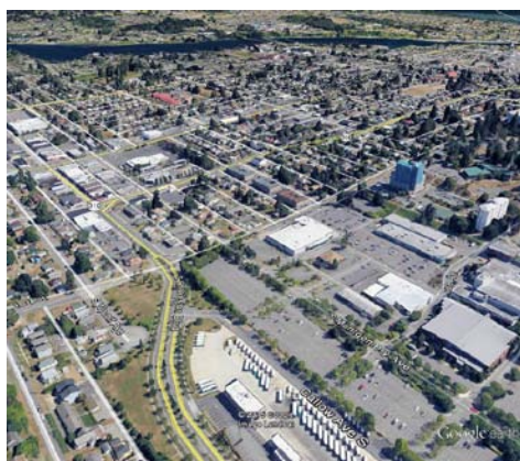
Figure 4.2.17. S Montgomery Avenue is a major utility corridor.
