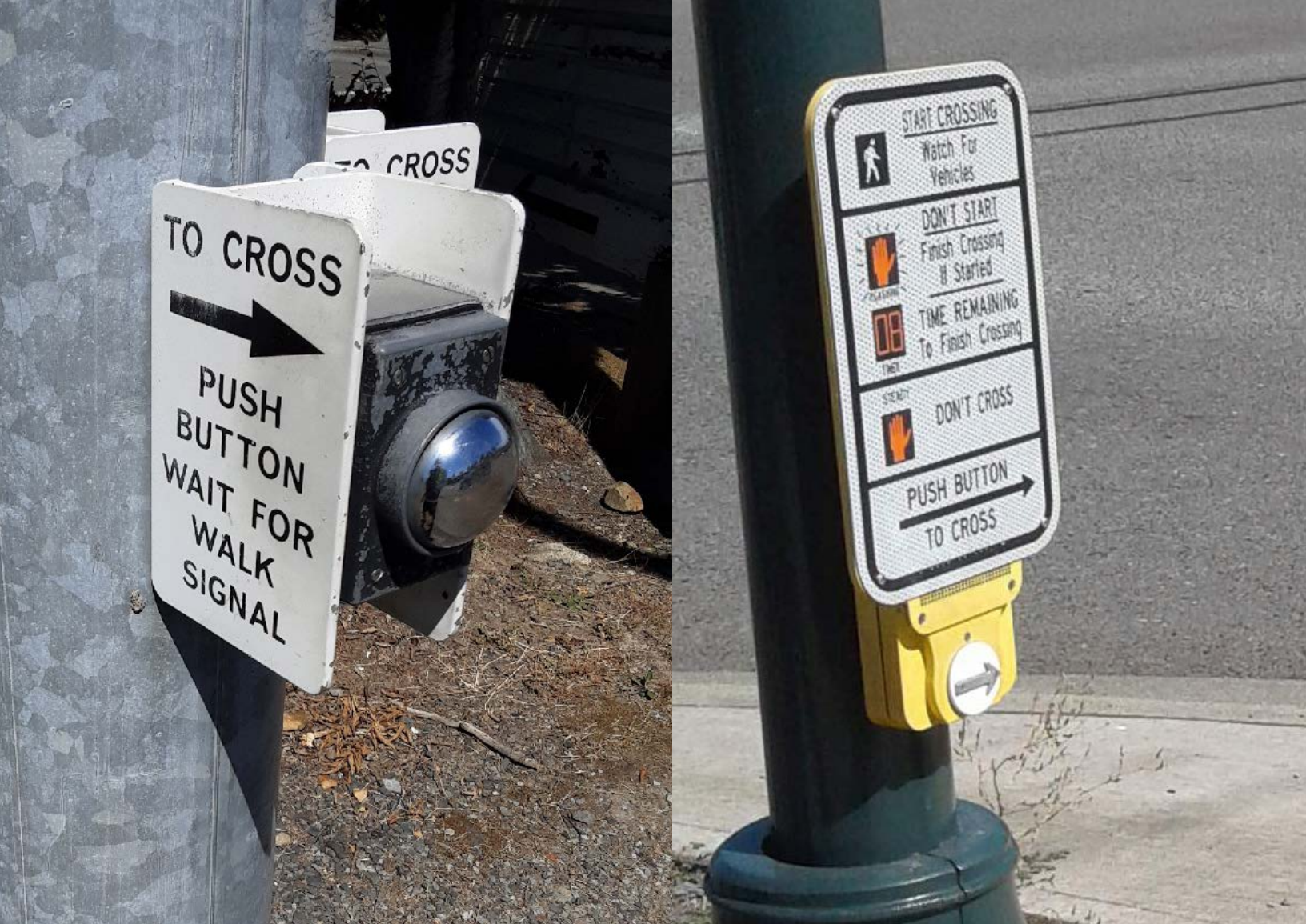
Figure 2.17 “H-style” And APS-style Pedestrian Push Button
