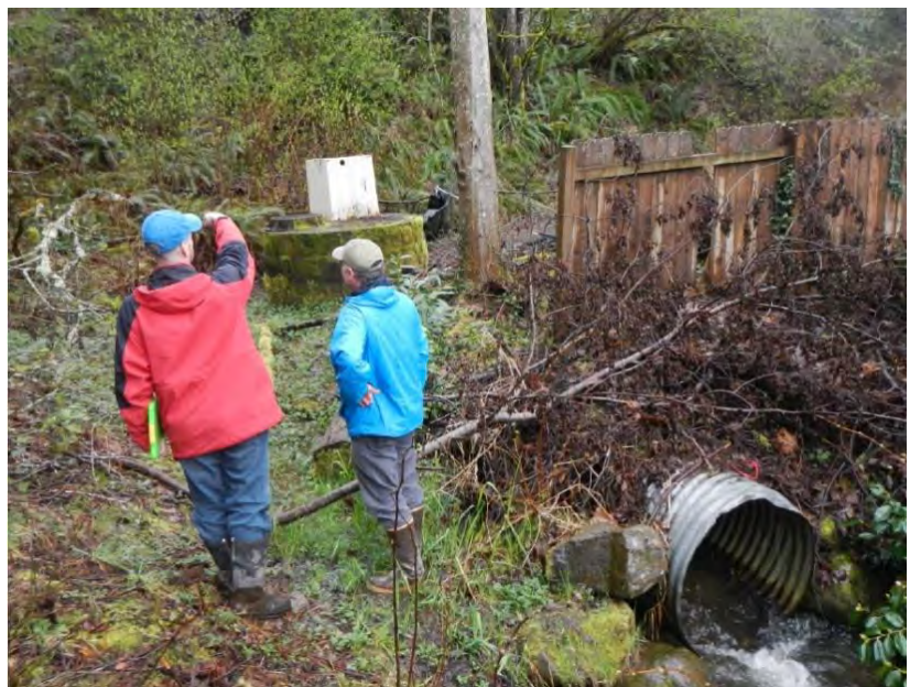
Photo 1: 36-inch CMP and control structure outfall downstream of Colchester Drive.
