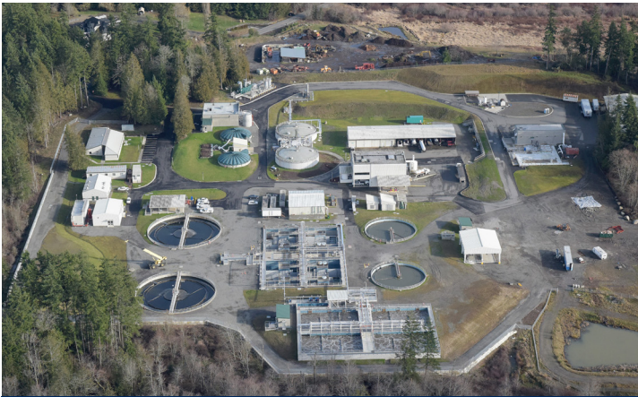
Aerial view of the Central Kitsap Wastewater Treatment Plant
