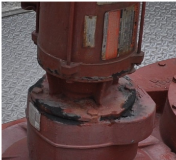
Grit Trap Corrosion around motor
