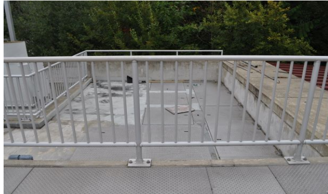
Headworks Aeration Channel and Flow Splitter
