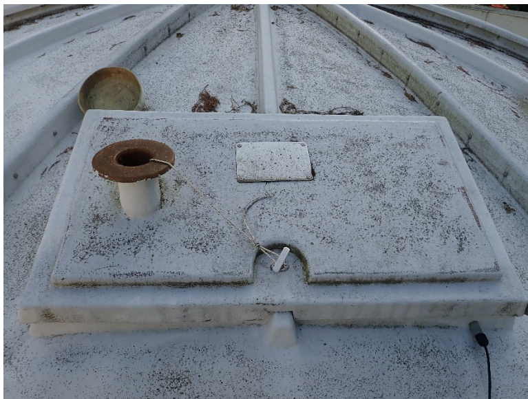
Figure 3-26. SWWTP sludge storage tank high-level switch installation
