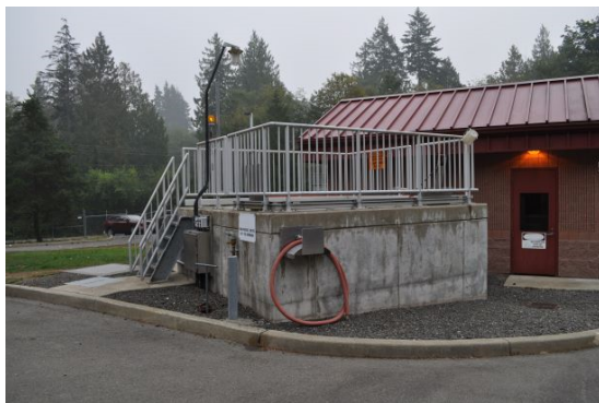
RAS PS and ML Splitter Box Structure
