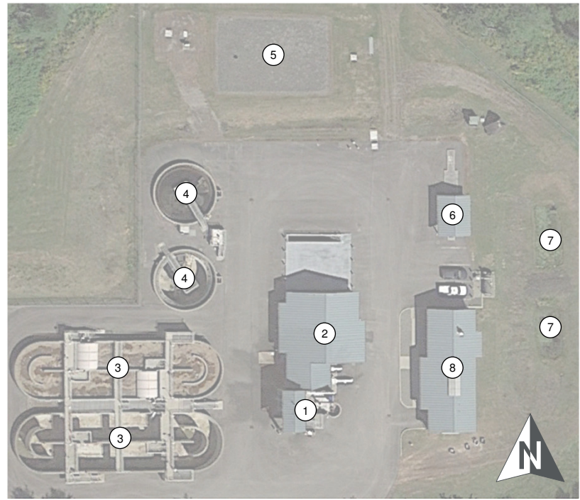
KINGSTON WASTEWATER TREATMENT PLANT
