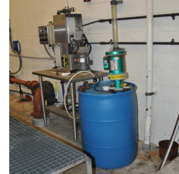
Polymer system for GBT
