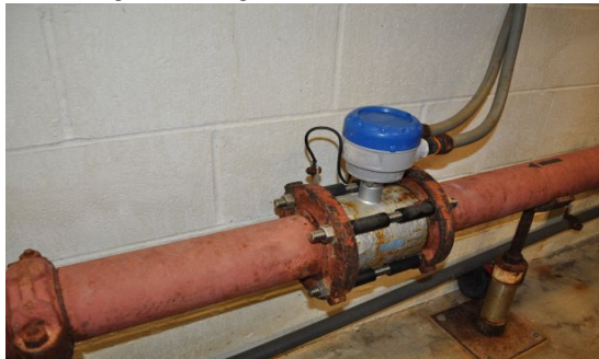
FE 606 Sludge to GBT Magmeter
