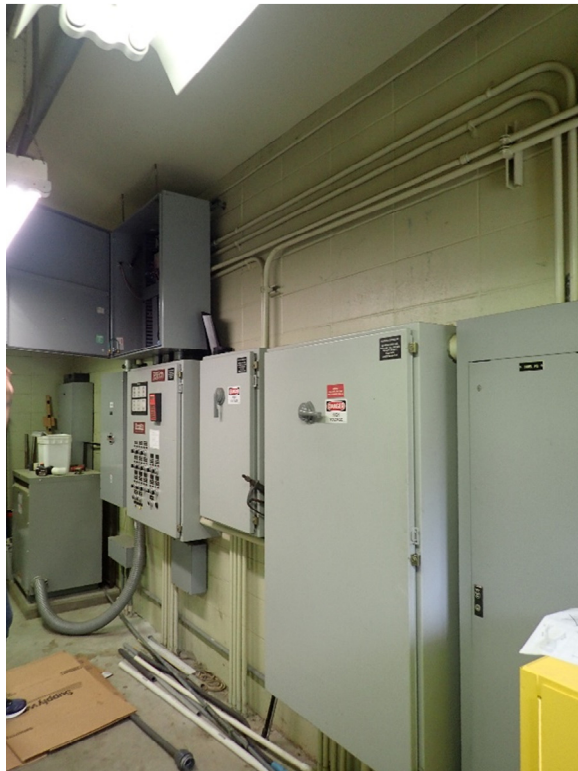
Figure 3-4. MWWTP blower building RIO control panel installation
