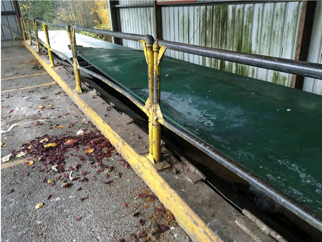
Figure 9: Hinged Sheet Steel Bridge Plates
