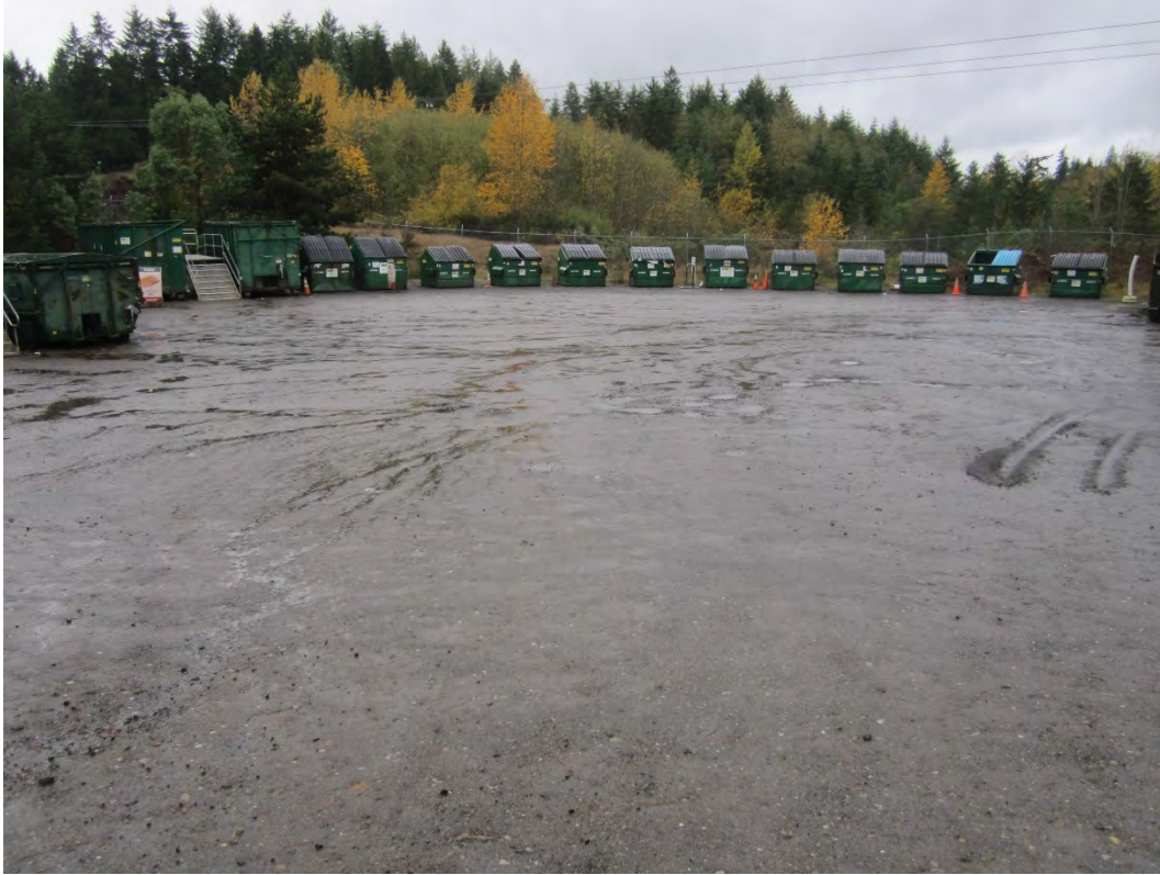
Figure 7. Existing Recycle Area
