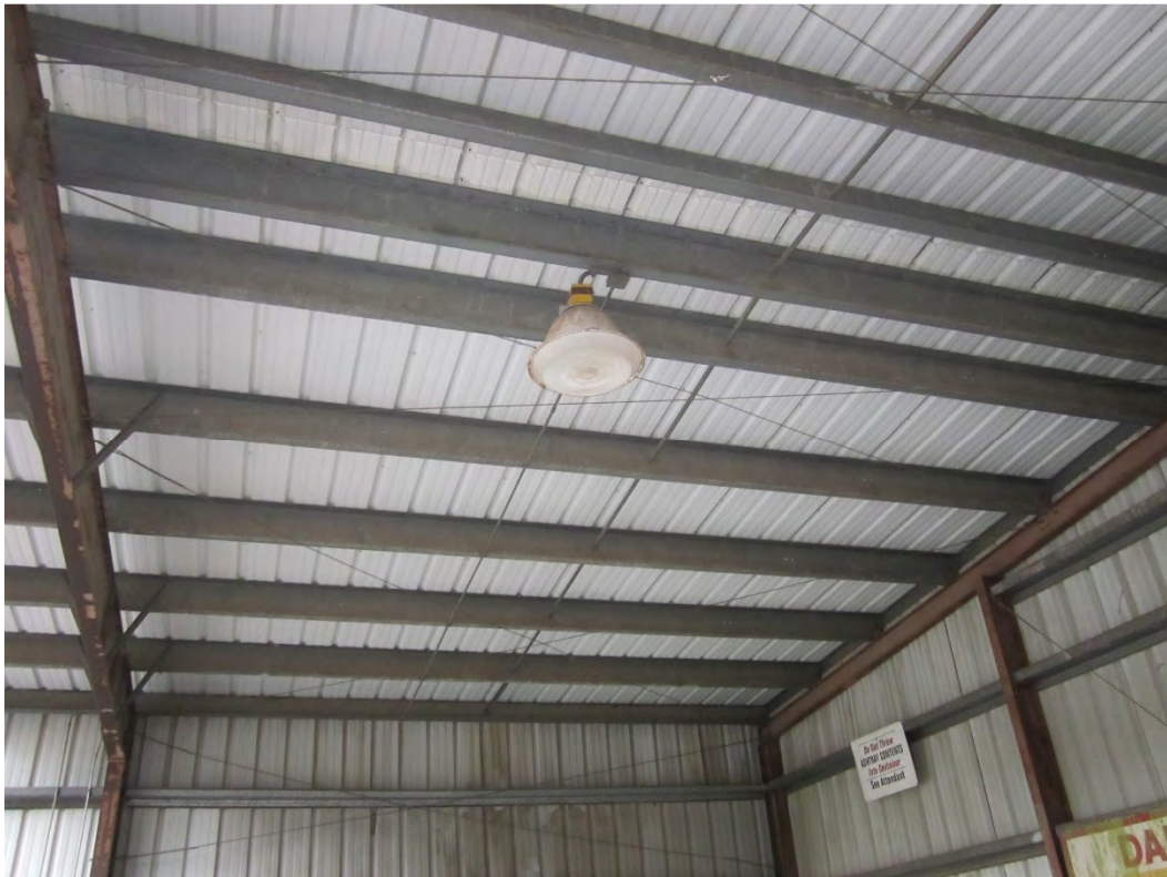
Figure 4: Center Hung HID High Bay Luminaire
