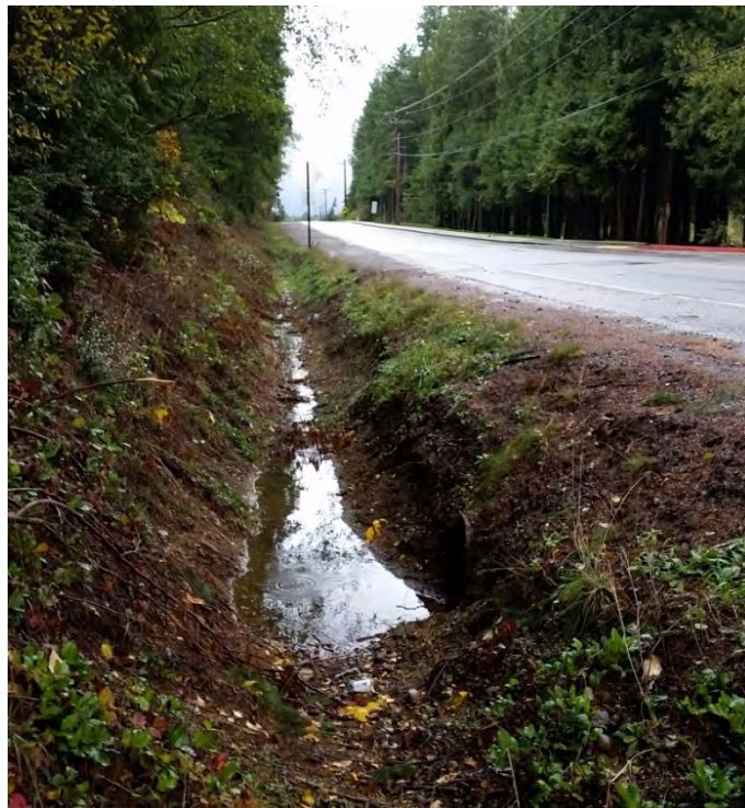
Figure 8: Photo Location 6 – Viewing North
