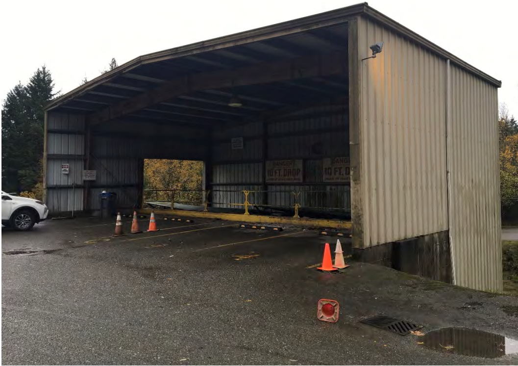
Figure 1: Refuse Shed C Unloading Area
