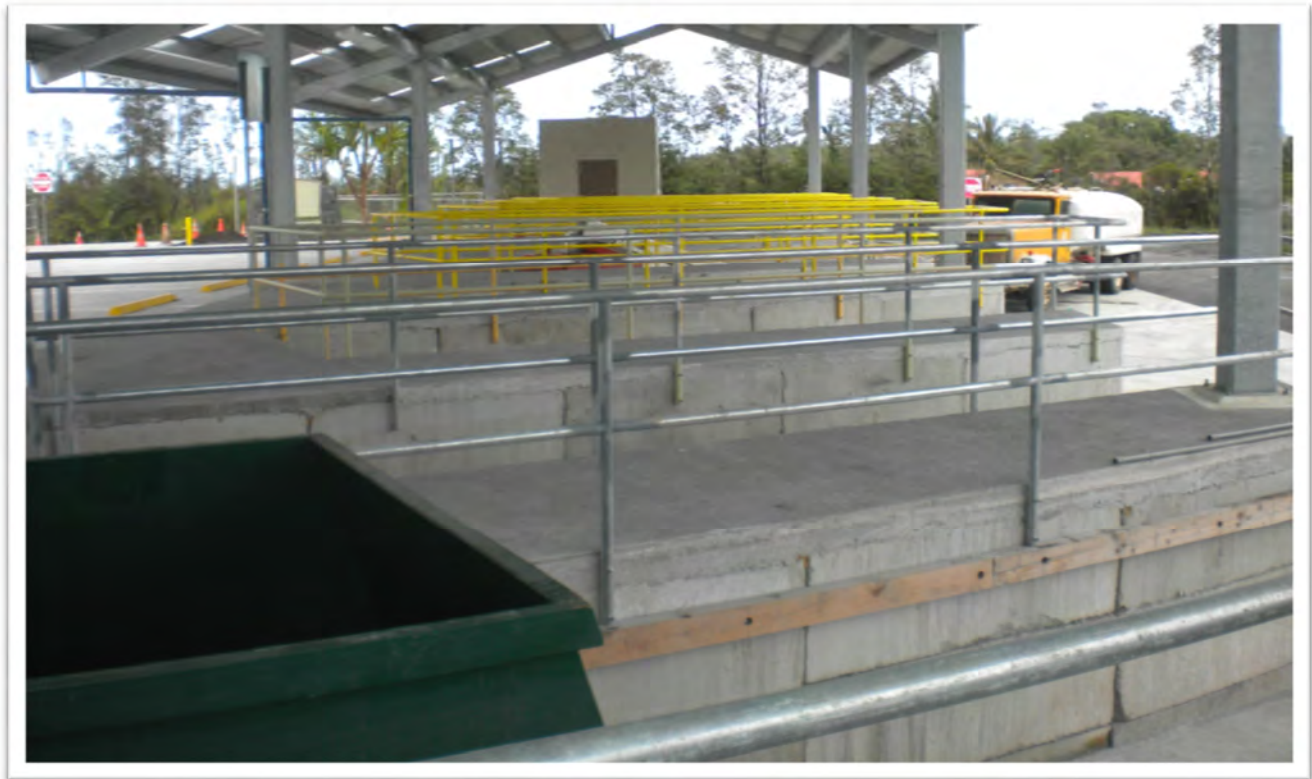
Figure 1: Example Finger Wall with Canopy
