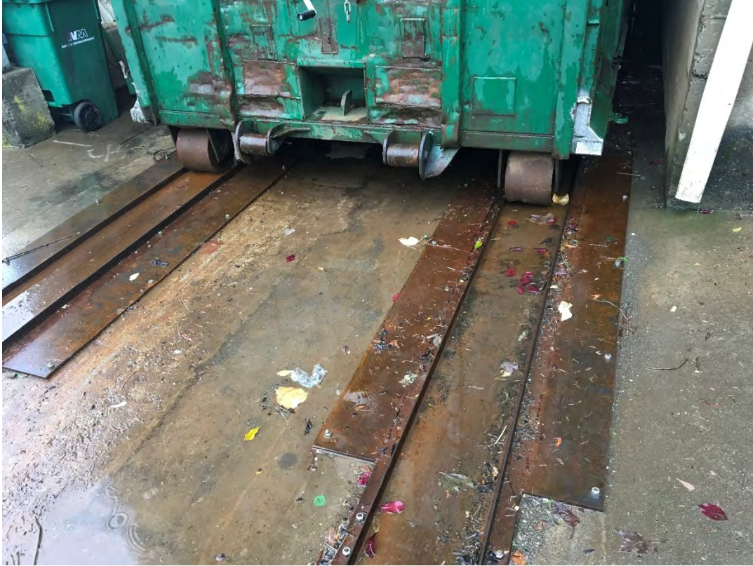
Figure 11: Surface-mounted C-channels on Steel Bridging Plates
