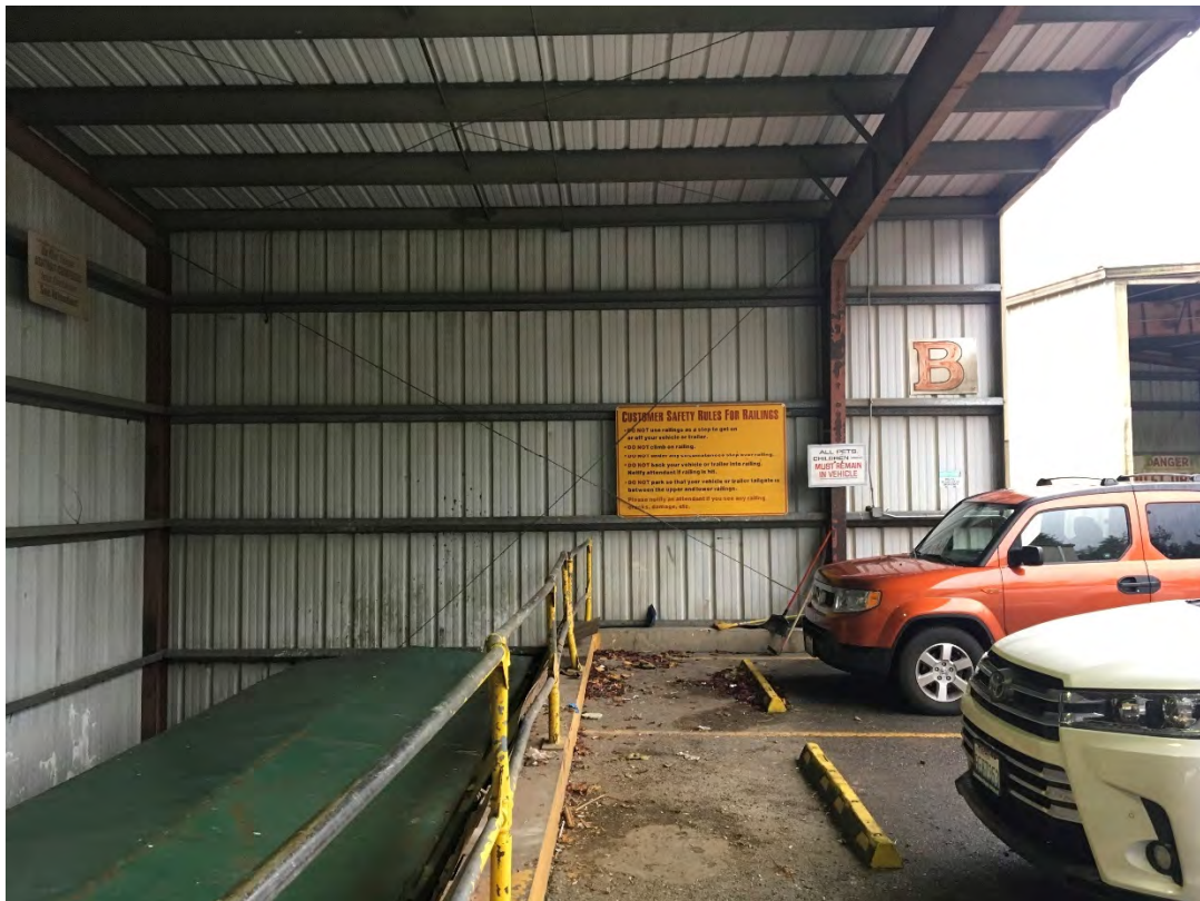
Figure 8: Two-rail Demountable Railing System
