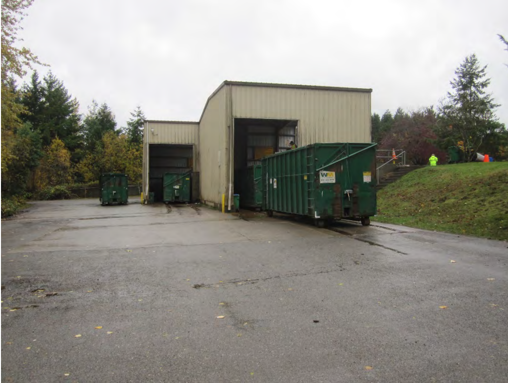
Figure 6. Existing Refuse Hauler Maneuvering Area
