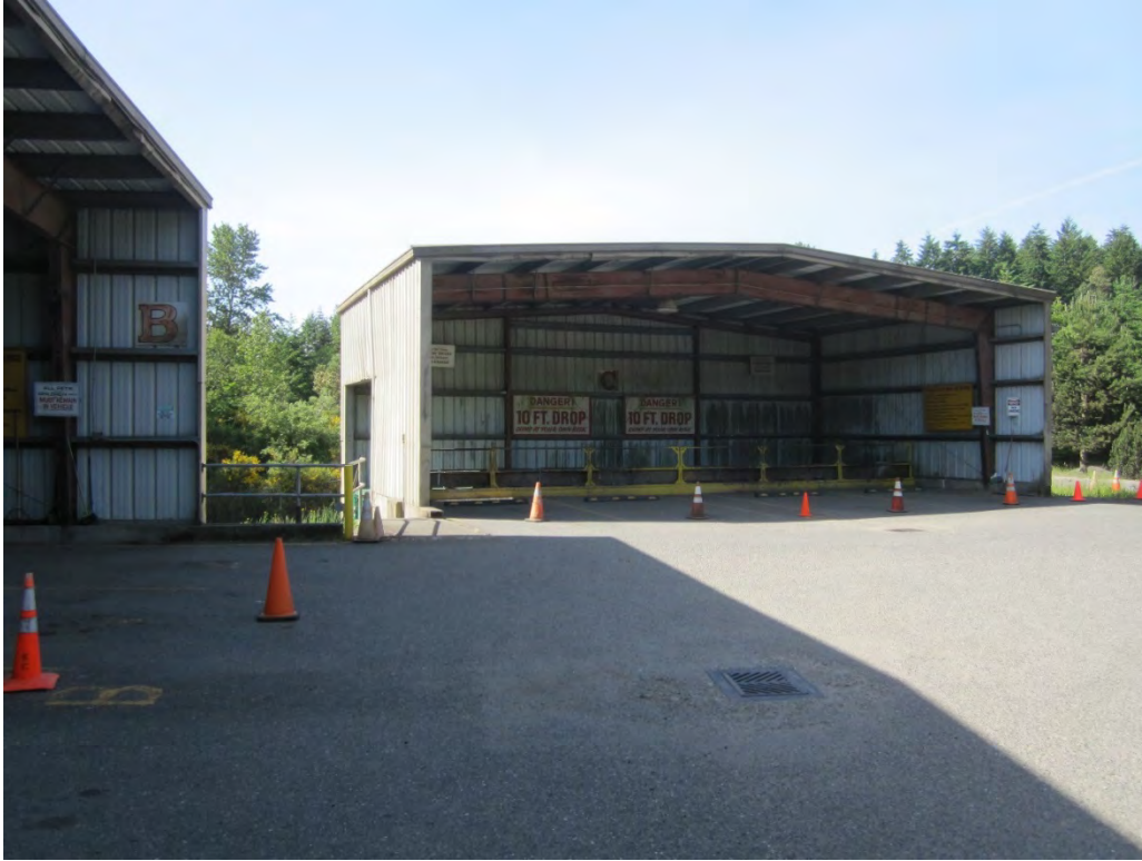
Figure 4. Existing Refuse Shed
