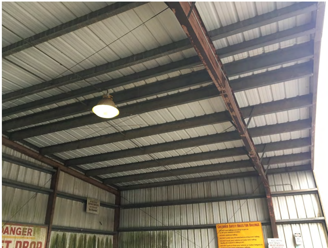
Figure 4: Clear-span Building Frame
