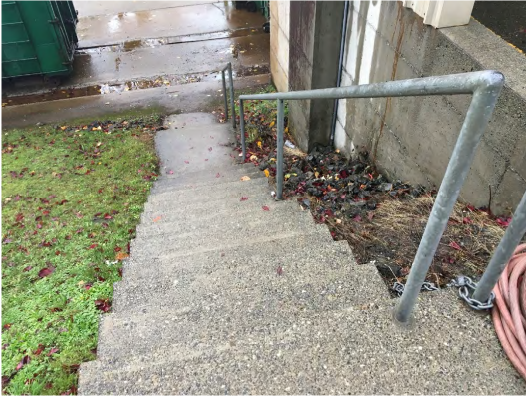
Figure 13: Concrete Stairs Fitted with Pipe-rail Handrails
