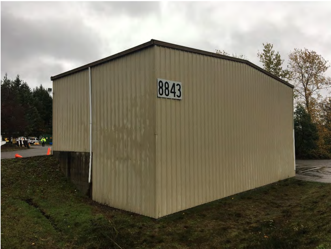
Figure 2: Refuse Shed C Exterior
